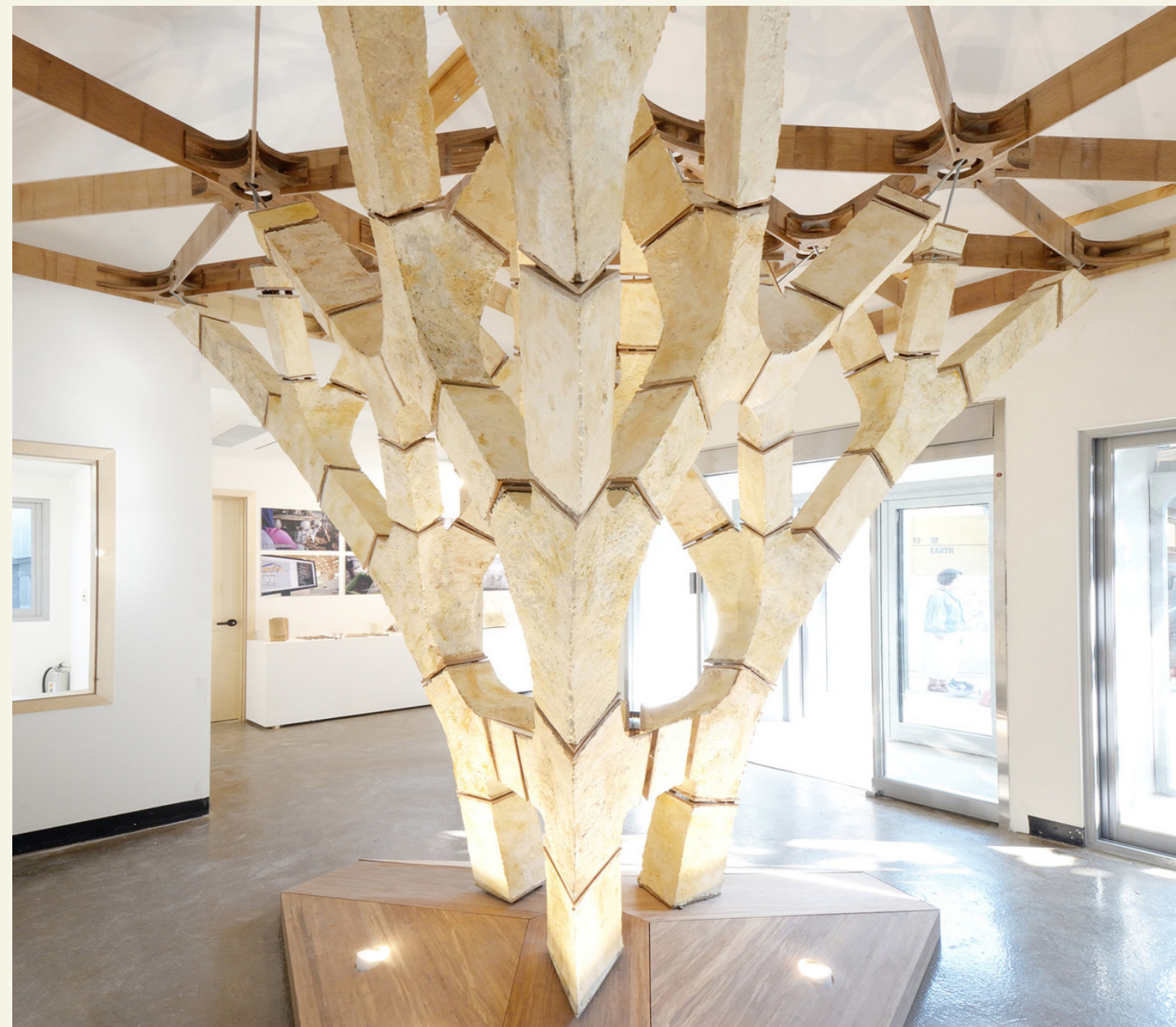
Bamboo and Jute Natural Fibre Reinforcement
